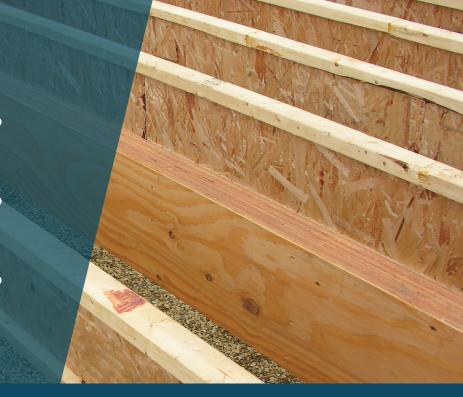
• P3 Joist of the same depth are manufactured with various flange widths; flange width is an important design consideration when specifying hangers.
