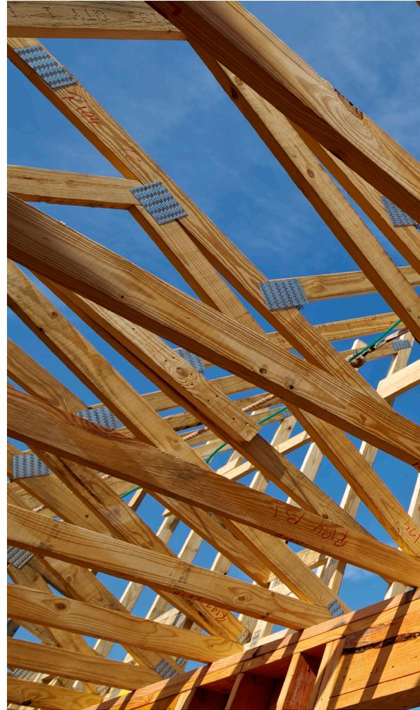
**Interfor SYP MSR 2400F** lumber is produced from our mills in Georgia. It offers the strength and stiffness ratings to meet the most demanding engineering applications in roof and floor trusses. Our SYP 2400F is available in 2x4 - 2x12, 8' -20'.
