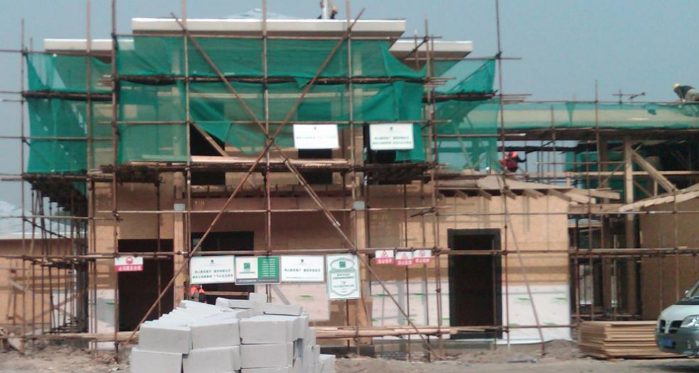
House framed with SPF lumber
