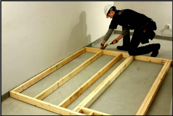
Apartment infill walls / partition walls
