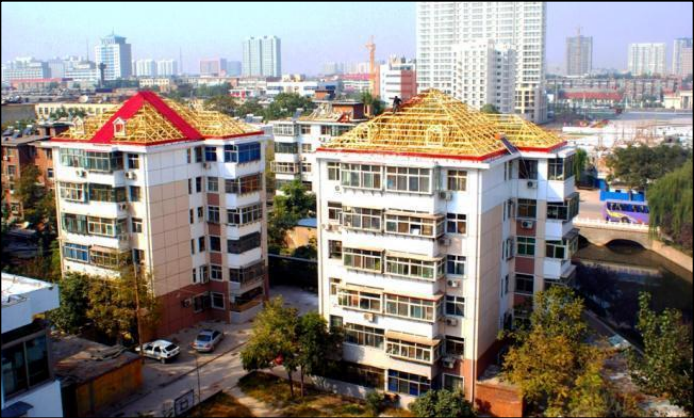
Wood truss re-roofing (east and north China)
