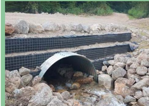
When Interfor builds forest roads, crossings on fish-bearing stream are designed to maintain fish habitat and ensure fish passage. This arch culvert has an open bottom, that maintains the original stream bed. Other design elements, such as the retaining wall and rock placed adjacent to the creek help prevent sediment from washing off the road surface and fill slopes and entering the creek.
